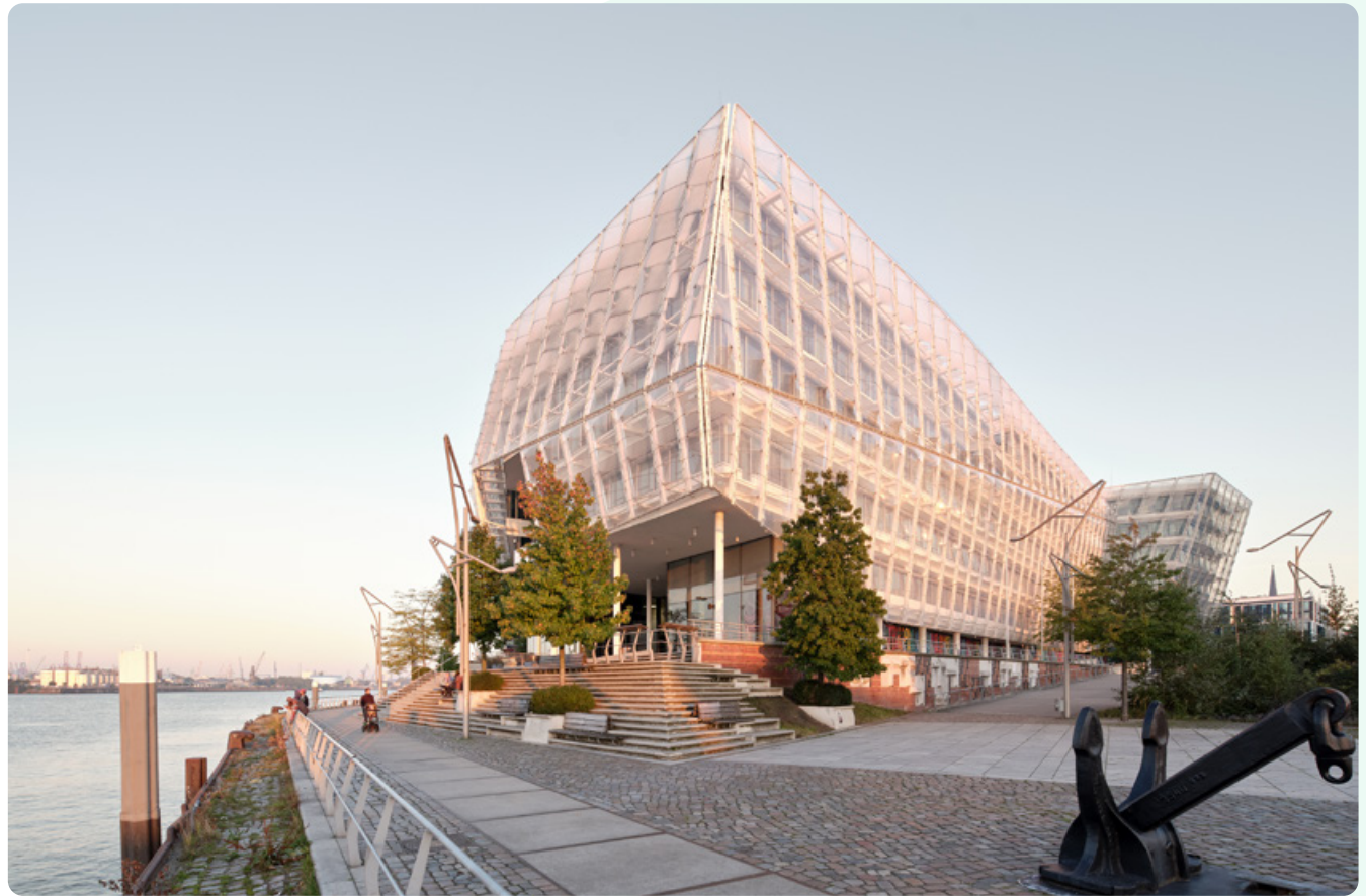
Hamburg corporate headquarters: "NEW WORK Harbour": Extensive controls and regulations guarantee a safe and correct working environment.
