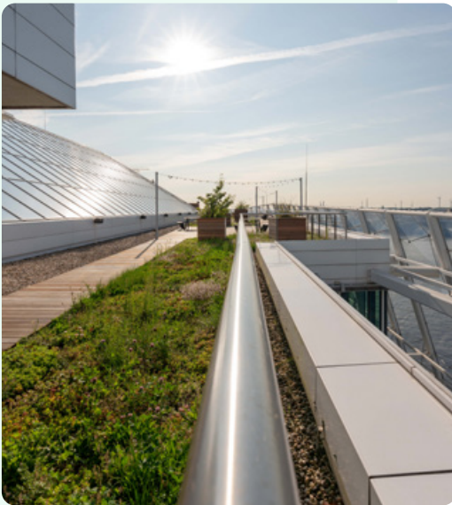
Green roof terrace of the NEW WORK Harbour: We want to reduce our emissions long-term.
